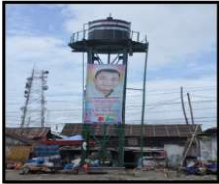
The Water Tank
