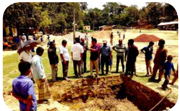
Citizen group orientation on Kalerpara UP office to Sonamoha Hut road construction under Dhunat upazila.
