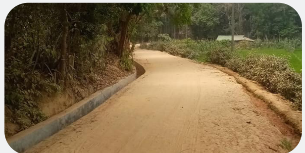
Construction of Chonkhola-Noapara road, P.M. Khali Union, Cox's Bazar sadar.
